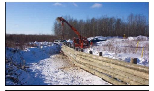
One of the three berms built to protect transmission line poles during breakup.
